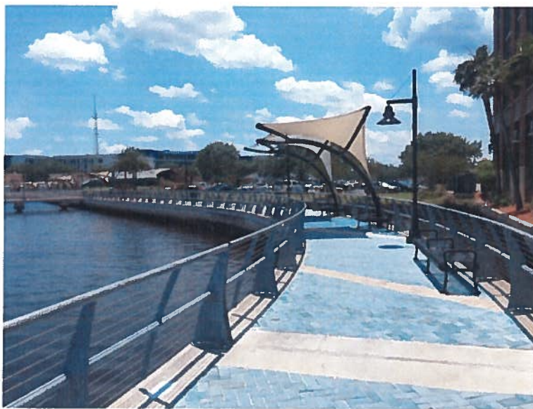
Existing Southbank Riverwalk railing and materials.
