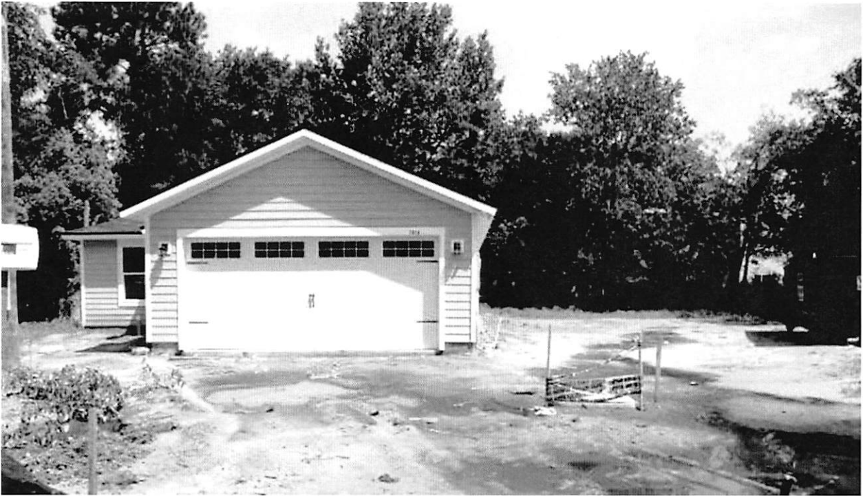
Dwelling under construction on a portion of the subject property
