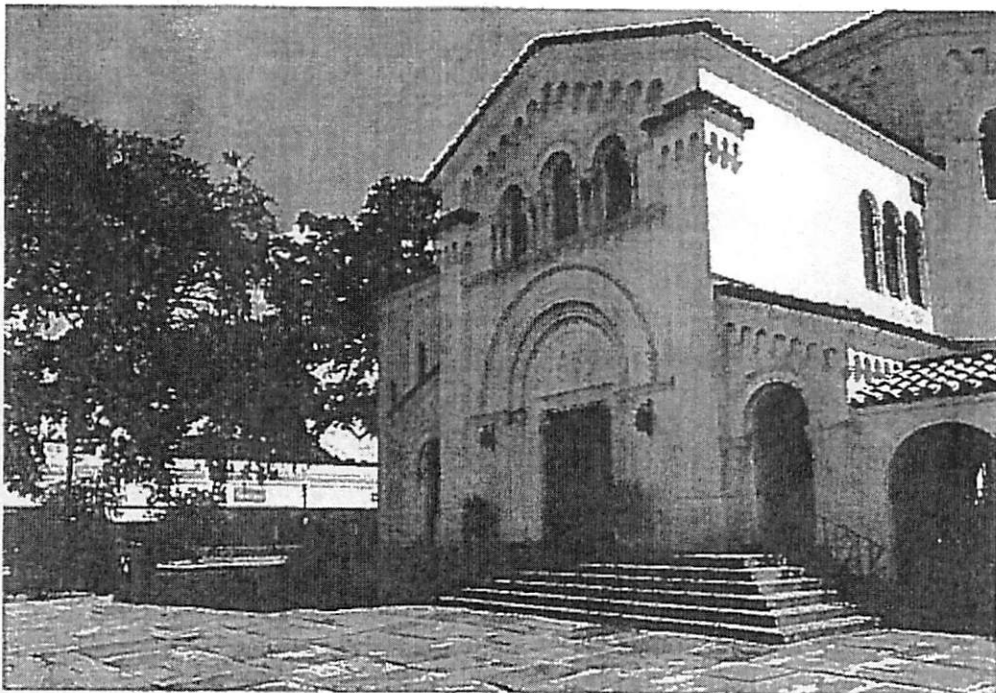
Property to the south: Church (2650 Park Street)
