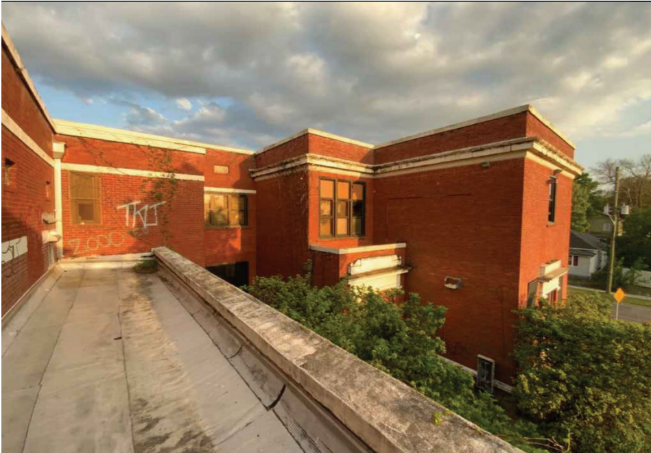
Exterior of building facing southeast
