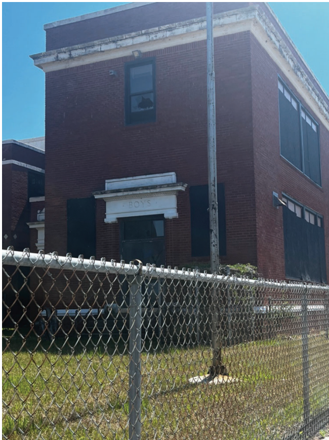
Southwest Corner Closeup
