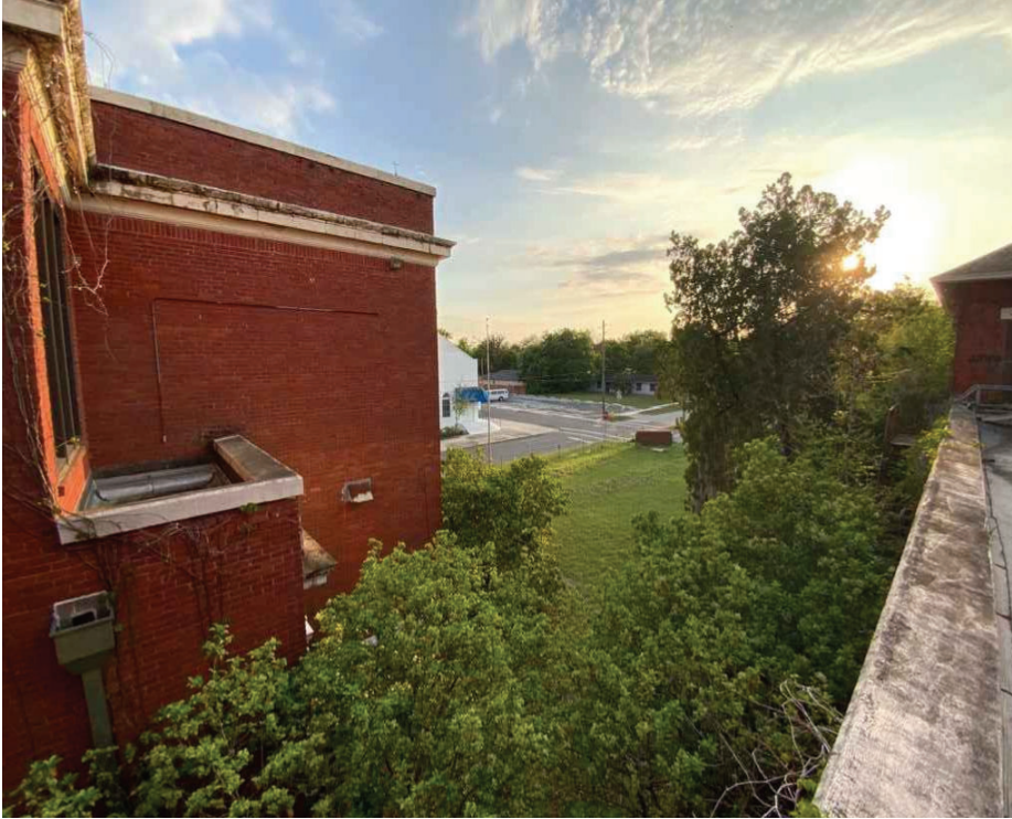
Exterior of building facing southwest
