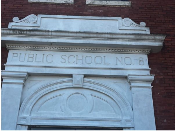
West Entrance Close up
