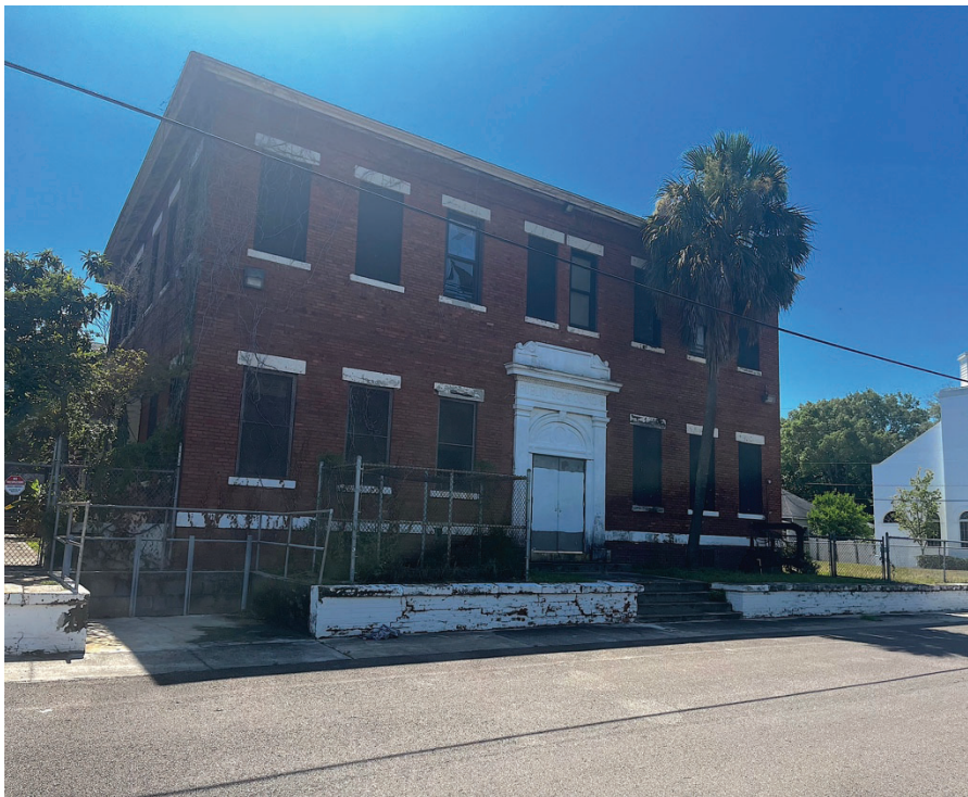
Front of Building – West Entrance
