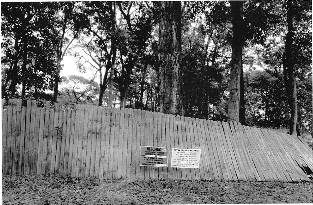
Source: City of Jacksonville Planning & Development Department, 01/26/2022 View of subject property from Whitlock Avenue.
