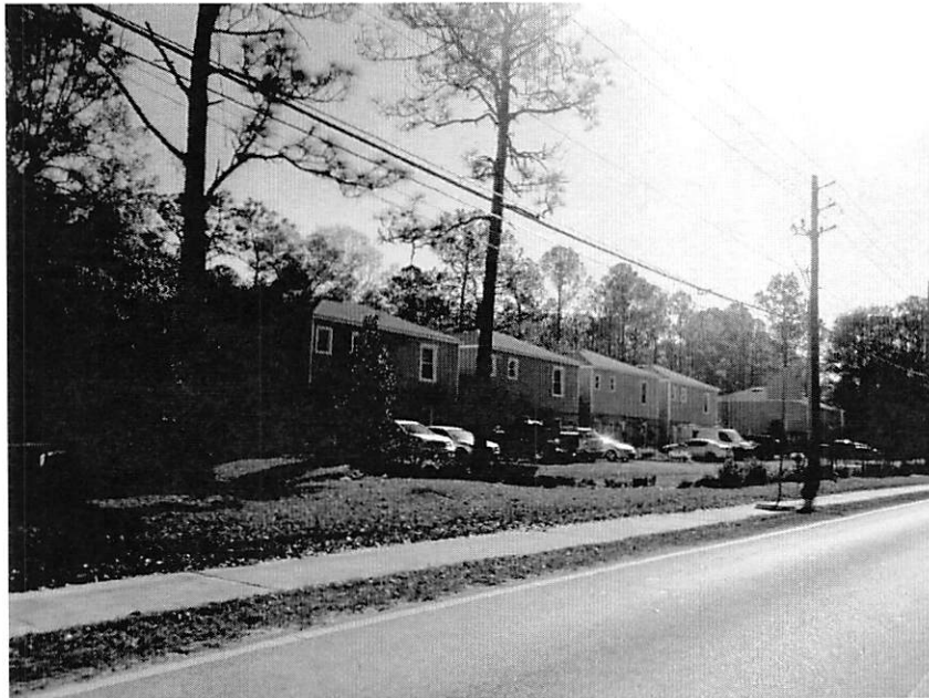
View of the Neighboring Multi-Family Dwellings
