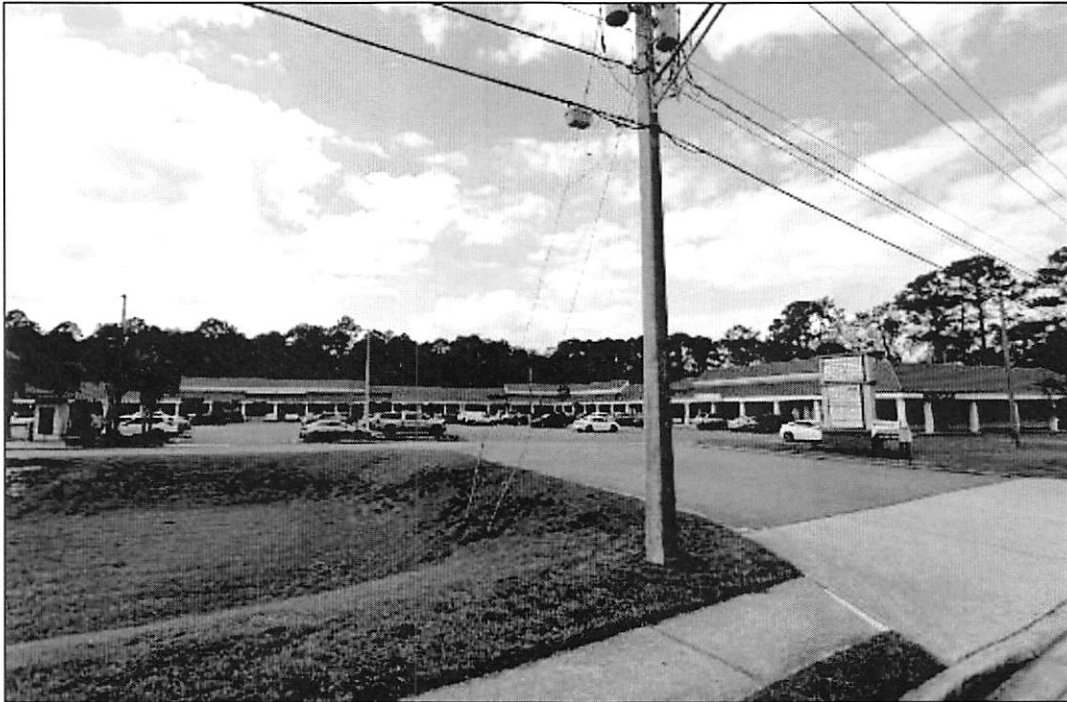
View of property to the West
