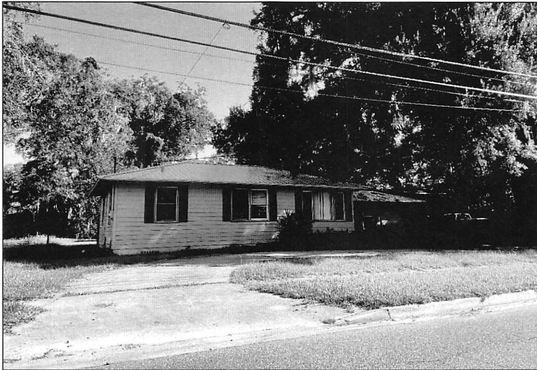
Property to the East (4817 Kingsbury St-75 Feet of Frontage)
