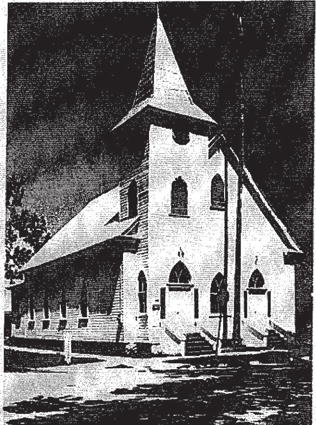
FE-12 ★★ PLEASANT GROVE PRIMITIVE BAPTIST CHURCH 740 VAN BUREN STREET DATE: ca. 1908-1909 ARCHITECT & BUILDER: Unknown
