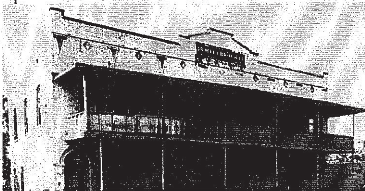
FE-11 ★ WELLBROCK BUILDING 606 EAST UNION STREET DATE: 1912 ARCHITECT: Wilbur B. Talley BUILDER: J. B. Cox
