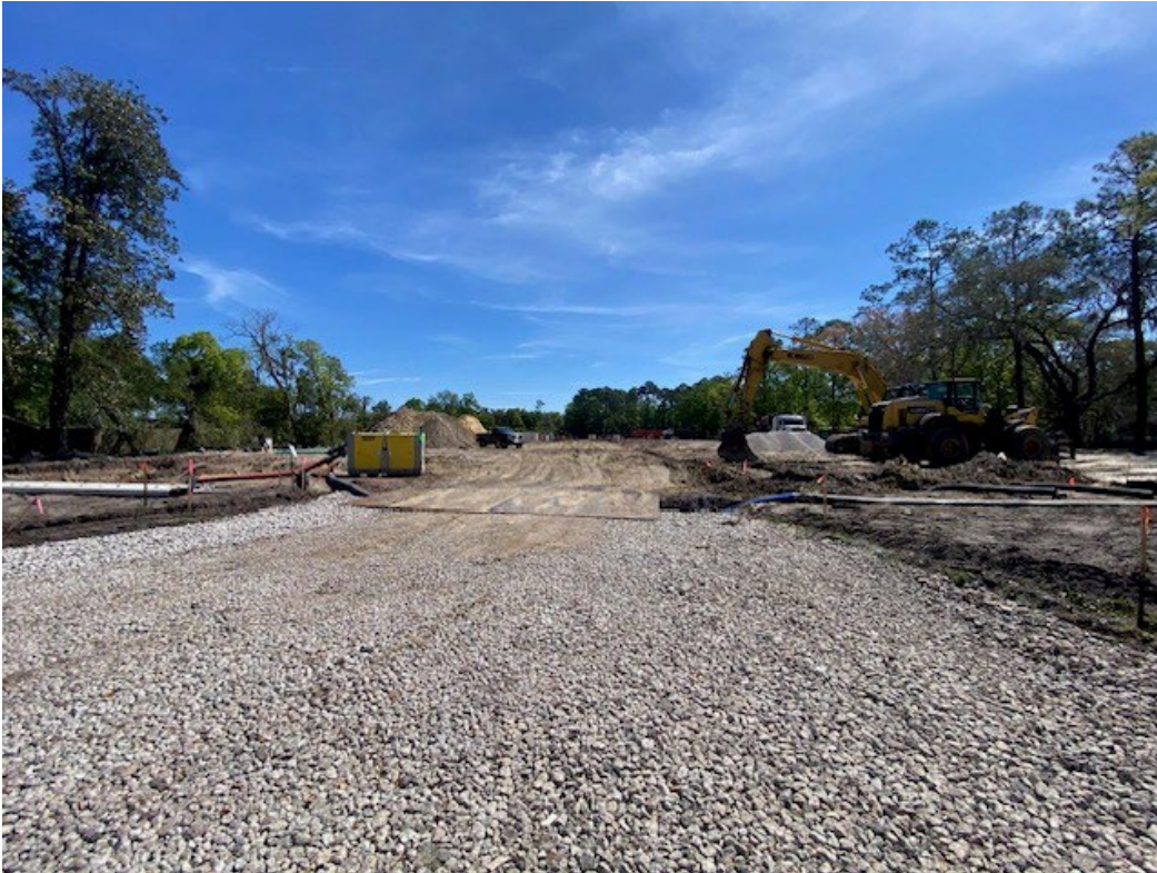
View of Subject Property from Camden Road.
