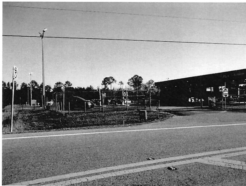
View of the Rental Car Facility
