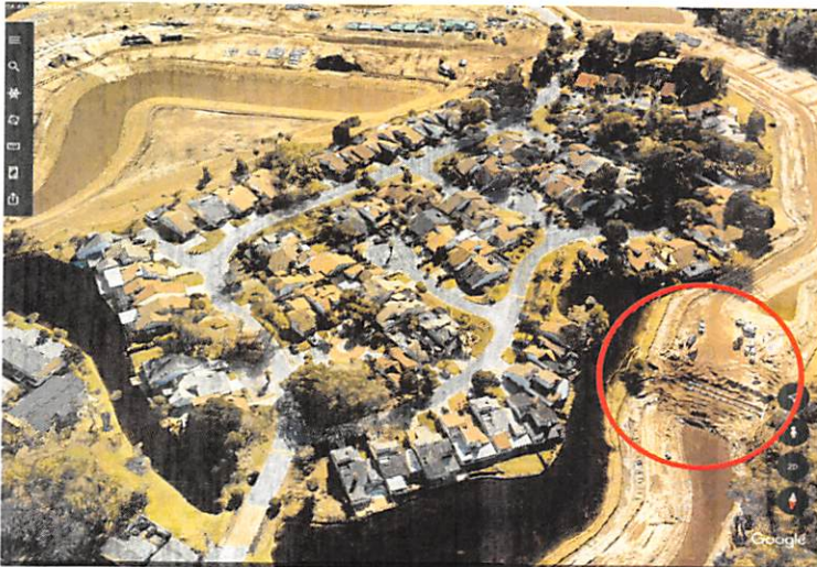
Photo 3: Stormwater measures to protect D.R. Horton new community, Meadow Walk (note red circle). Resolves issue with Zone 2 (map).
